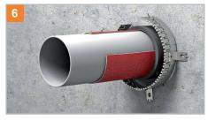
Bend two lugs on one end of the metal wrap by  $90^\circ$  so that both ends will connect. Insert the bended lugs into the horizontal openings. Finally, bend the lugs again so that the collar is closed tightly.
